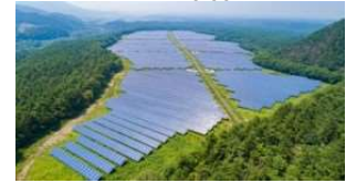
S-17 CS Daisen-cho Power Plant (A)(B) 27.3MW
