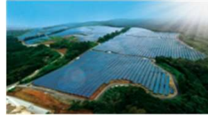
S-13 CS Mashiki-machi Power Plant 47.7MW
