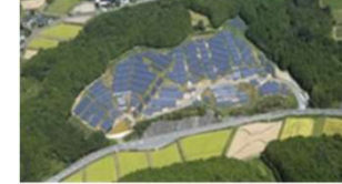
S-15 CS Tsuyama-shi Power Plant 2.0MW
