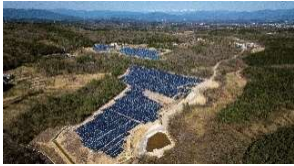
S-16 CS Ena-shi Power Plant 2.1MW
