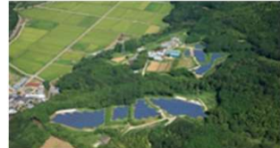
S-12 CS Kannami-cho Power Plant 1.3MW
